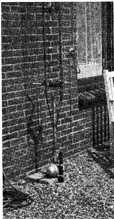
The VHF aerial system at PA0FB is supported by two towers of light alloy, which are extendable and rotatable; the base of each mast stands on a reversible motor, as can be seen in this photograph, which also shows the extension winch.
